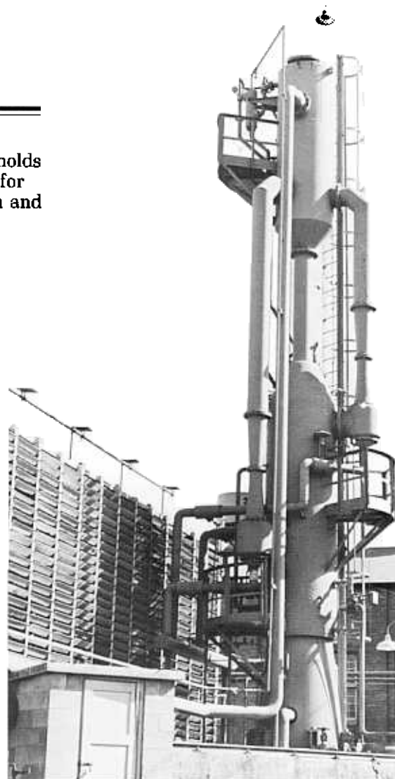
200 ton C-R CHILL VACTOR steam jet refrigeration unit chills water for bleaching operations at Crown-Zellerbach Corp.
