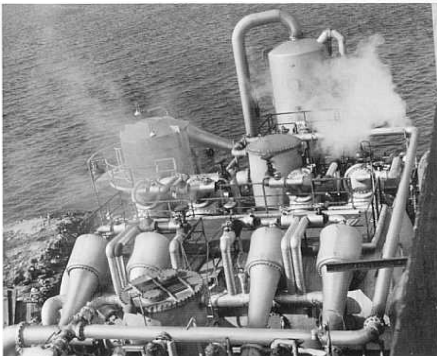
The largest producer of antibiotics in the United States uses this CHILL-VACTOR to chill 12,000 gallons of process water per minute. The photograph shows only a portion of the large and complex installation.
